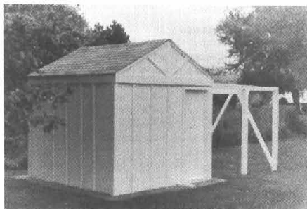
Figure 3. Rolling Ridge Observatory as it sits in my backyard. The peaked roof design was selected to accommodate snow loadings and to complement other structures in the neighborhood.
