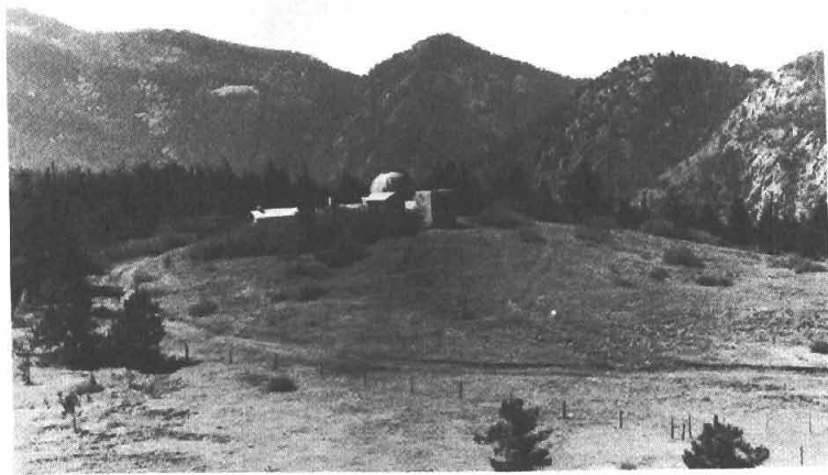
Fig. 1. View toward southeast of Capilla Peak Observatory complex.
